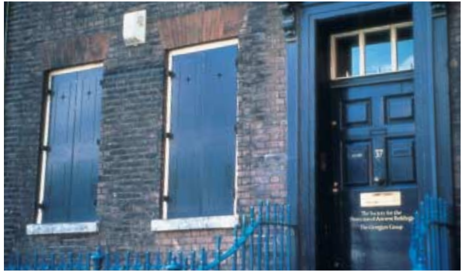
Figure 10 Shutters are not just historically important, they can provide significant thermal improvements as well as enhanced security and reduction of dust and noise. (Photograph: (b) courtesy of Matthew Slocombe and the Society for the Protection of Ancient Buildings; (a), (c), (d) and (e) by Chris Wood and other members of English Heritage Building Conservation and Research Team)
