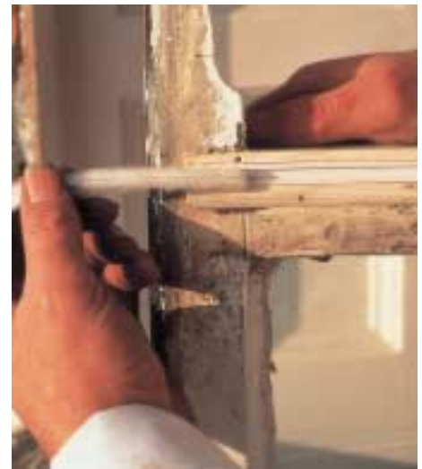
Figure 8 Draughtproofing strip being inserted into a routed channel on the bottom rail of the top sash. (Photograph courtesy of Ventrolla Ltd)
