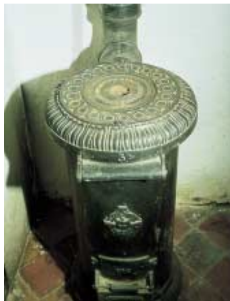
Figure 15 Examples of early cast iron stove and radiator which are still in use. Items such as these should continue to be used and if necessary refurbished to improve efficiency. (Photograph of stove courtesy of Robyn Pender; photograph of radiator by Chris Wood)
