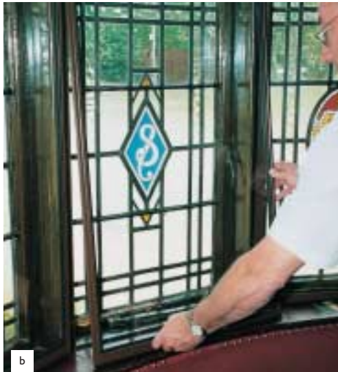
Figure 16 The heat loss from this listed public house has been dramatically reduced by the installation of discreet secondary glazing (b) and (c). The glazed panels can be easily removed in summer. (Photographs courtesy of Storm Windows, Leeds, © copyright Storm Windows, Leeds)
